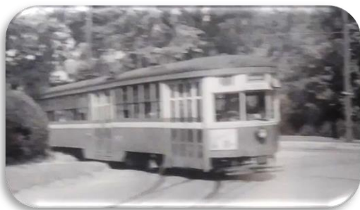
Car 707, on its way west to Woodbine and Magnolia, squeals around the tight turn from Fillmore onto Washington in Kirkwood shortly before the line closed in August 1950.
